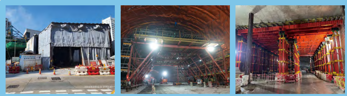
甘肅街的隔音罩 Noise enclosure at Kansu Street 襯砌隧道 Construction of tunnel lining 建造近新碼頭街的馬頭角明挖回填隧道 Construction of Ma Tau Kok cut-and-cover tunnel near San Ma Tau Street
