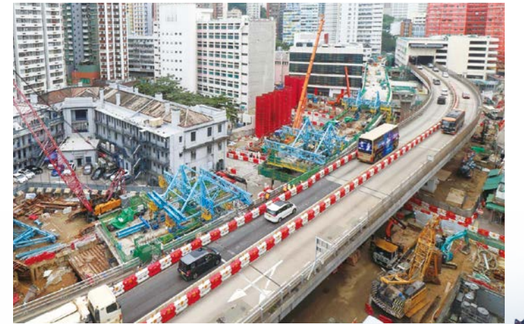
加士居道天橋重置工程採用「移動模板」及「就地澆築平衡懸臂法」 "Cast in-situ balanced cantilever method with Form Traveller system" has been adopted for the re-provisioning of the GRF
