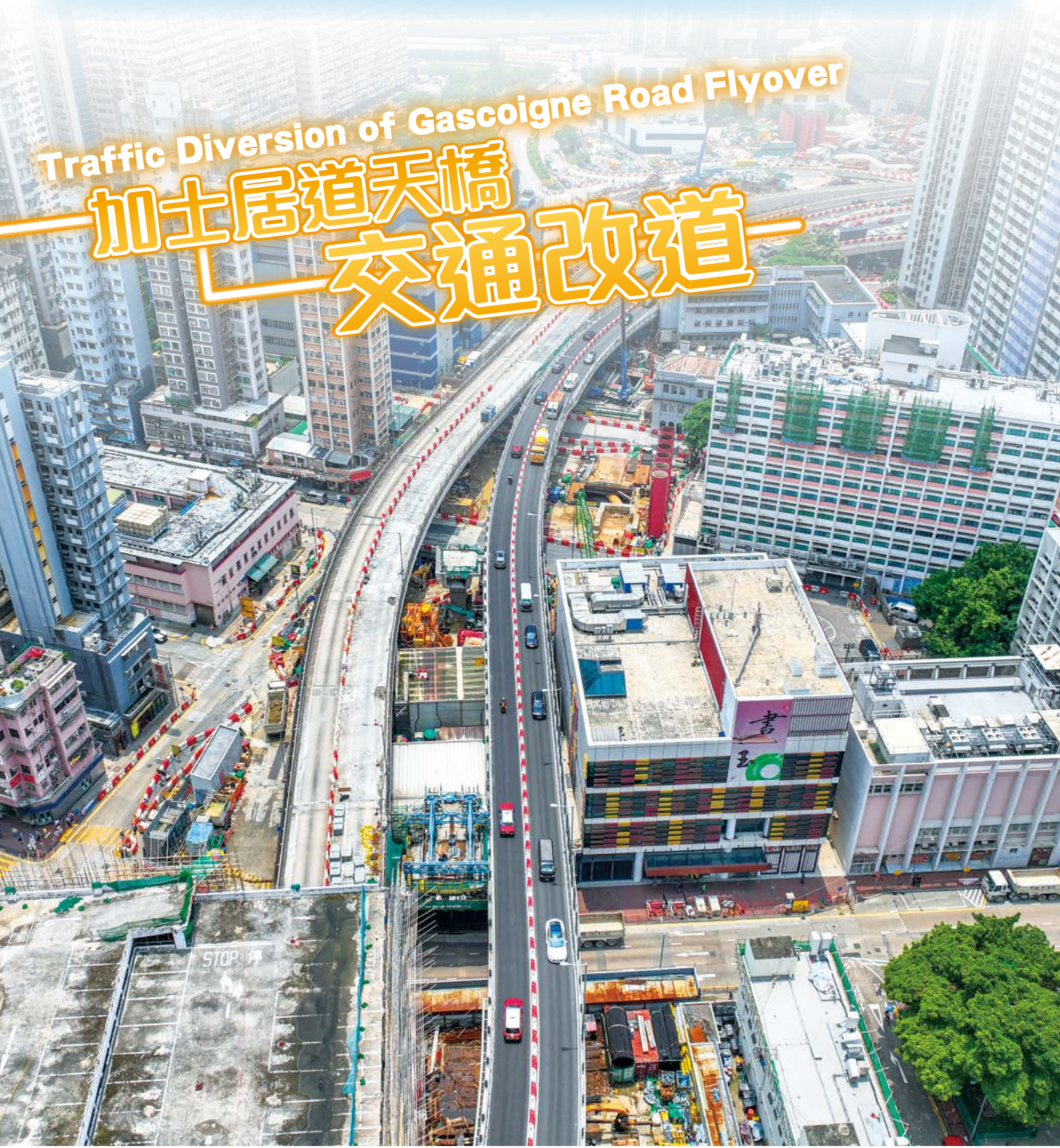
現時加士居道行人天橋 Existing GRF 加士居道天橋交通已改道至重置的一段行人天橋 Traffic from GRF has been diverted to a section of re-provisioned flyover 重置的行人天橋 (北面部份) Re-provisioned flyover (northern section)
