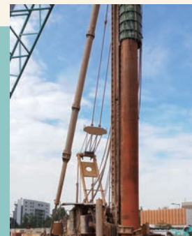
海泓道工地的園景平台鑽樁工程 Piling works for landscaped deck at Hoi Wang Road works site
