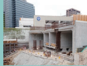
麗翔道工地的通風坑道的建造工程 Construction of ventilation adit at Lai Cheung Road works site
