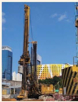
啟德通風大樓及行政大樓的嵌岩鋼工字樁安裝工程 Pre-bored socketed H-pile installation works at Kai Tak Ventilation Building and Administration Building works site
