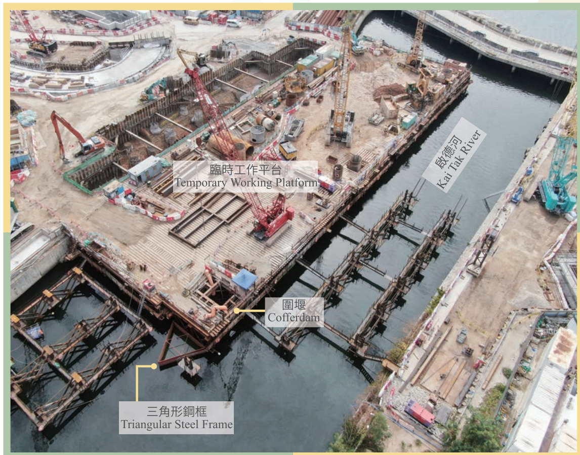
橫跨啟德河的臨時工作平台概覽 Overview of temporary working platform across Kai Tak River
