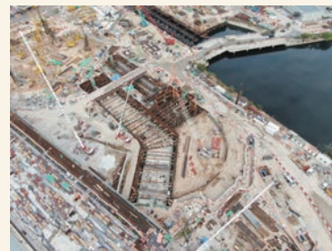
地下行車道、通風及機電坑道的結構建造工程 Construction of underpasses, ventilation and electrical and mechanical adit
