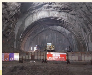
於何文田豎井通道工地的隧道鑽爆工程 Drill-and-blast works at Ho Man Tin access shaft works site
