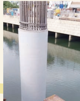
橫跨啟德河行車天橋的橋墩建造工程 Pier construction works for vehicular bridges across Kai Tak River
