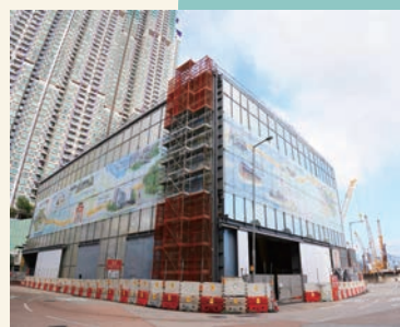
於馬頭角豎井通道工地興建的臨時隔音罩工程完成 Construction of temporary noise enclosure at Ma Tau Kok access shaft works site has been completed
