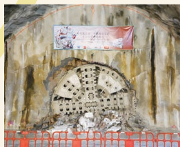
隧道鑽爆機已於2022年1月6日貫通先導隧道 TBM breakthrough the pilot tunnel was completed on 6 January 2022
