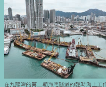
在九龍灣的第二期海底隧道的臨時海上工作平台及圍堰建造工程 Installation of temporary marine platform and construction of cofferdam for Stage 2 Underwater Tunnel at Kowloon Bay
