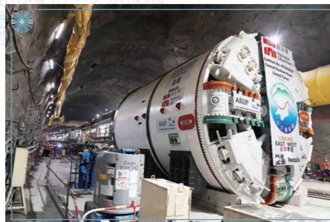
於隧道內組裝隧道鑽挖機 Assembly of TBM inside the tunnel
