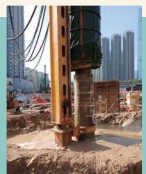
圍景平台的鑽樁工程 Piling works for landscaped deck
