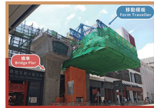
安裝移動模板後的重置加士居道天橋 RGRF after installation of Form Traveller
