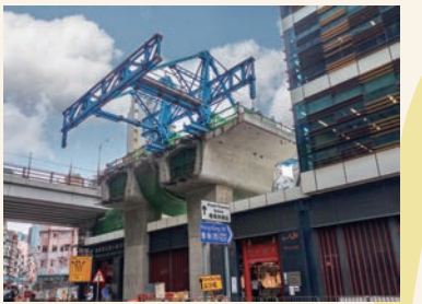
重置加士居道天橋工程 Reprovisioning of Gascoigne Road Flyover
