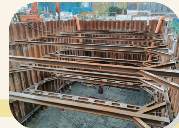
地下行車道和通風及機電管道的挖掘及安裝橫向支撐架工程 Excavation and installation of lateral support for underpass and ventilation and E&M adit
