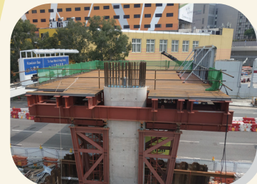
啟福道行人天橋臨時支撐架建造工程 Installation of temporary falsework for Kai Fuk Road Footbridge
