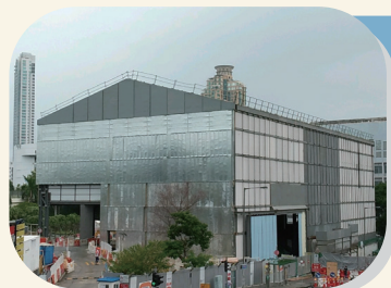
臨時隔音罩建造工程 Construction of temporary noise enclosures
