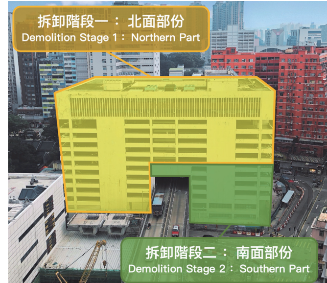
油麻地停車場大廈的拆卸安排 Demolition arrangement of the Yau Ma Tei Carpark Building
