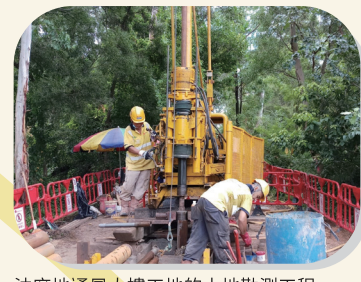
油麻地通風大樓工地的土地勘測工程 Ground investigation works at Yau Ma Tei Ventilation Building site
