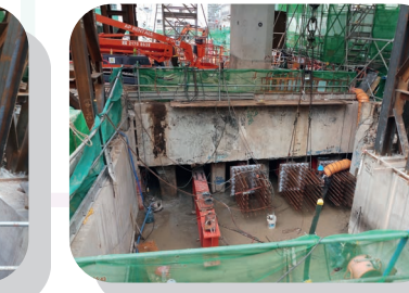
於地基樁帽下滑入大型鋼樑 Install large-sized structural steel beams underneath pile cap
