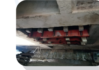
已切斷及分離的地基樁柱 Piles cut and removed
