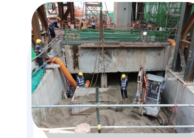
於地基樁帽下挖掘 Excavate underneath pile cap
