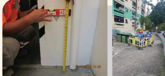
安裝監測點 Installation of monitoring points
