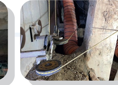
將地基樁柱切斷 Saw cut the piles
