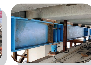
於加士居道天橋橋身底部安裝液壓千斤頂 Install hydraulic jacks at the soffit of GRF
