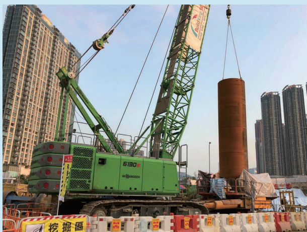
海泓道進行鑽樁工程 Bored piling works for Ventilation Adit at Hoi Wang Road
