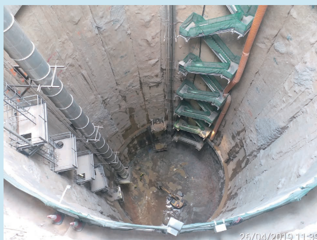
豎井通道挖掘 Access shaft excavation
