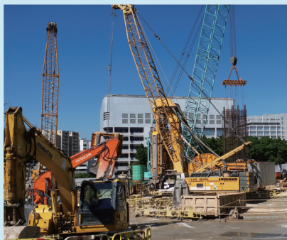
豎井隔牆建造工程 Construction of diaphragm wall for the access shaft
