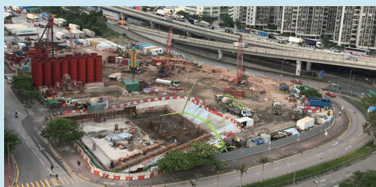
友翔道工地的隔牆建築工程 Diaphragm wall construction works at Yan Cheung Road works site
