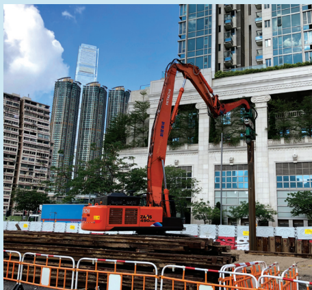
位於欣翔道的臨時母嬰健康院正進行板樁工程 Sheet piling works for the Temporary Yau Ma Tei Maternal and Child Health Centre located at Yan Cheung Road near Yau Cheung Road
