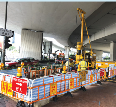
在油蔴地警署附近進行土地勘測工作 Ground investigation works near the Yau Ma Tei Police Station
