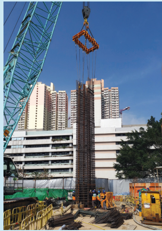
豎井連續牆建造工程 Construction of diaphragm wall for the access shaft
