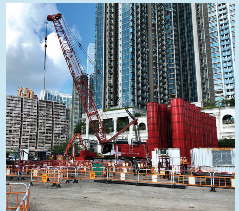
在友翔道為以明挖回填方式興建的隧道進行相關連續牆工程 Construction of diaphragm wall for the cut-and-cover tunnel near Yau Cheung Road
