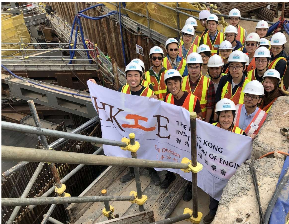
Members of HKIE Civil Division have a better understanding of the construction method of Cut-and-Cover Tunnel after the site visit at Kai Tak. 香港工程師學會土木分部的會員參觀啟德工地後，對明挖回填式隧道的建造方法有更深入了解。
