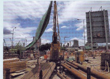
Pre-drilling works for vehicular bridges at Kai Cheung Road U-turn slip road
