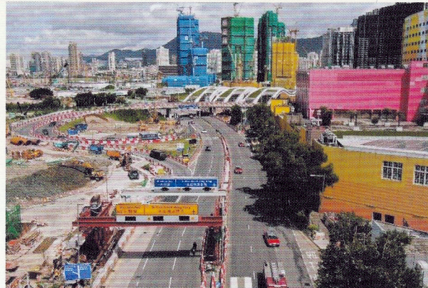
Temporary falsework for construction of Kai Fuk Road footbridge
