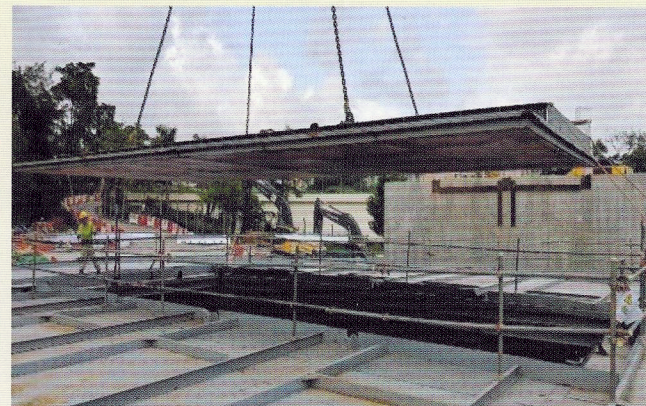
Access shaft was covered by noise enclosure
