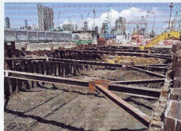
Excavation and installation of lateral for underpass
