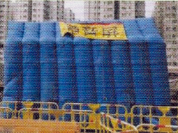
Erection of inflatable noise barrier
