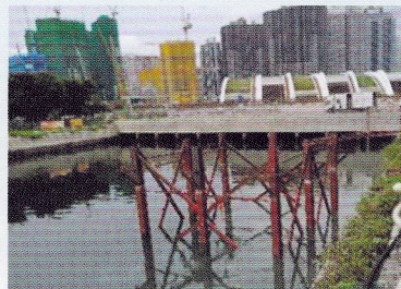
Installation of temporary platform for piling works across Kai Tak River
