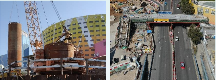
Bored piling works for vehicular bridges near Kai Cheung Road U-turn slip road Construction of bridge deck, staircases and lift shafts of Kai Fuk Road Footbridge
