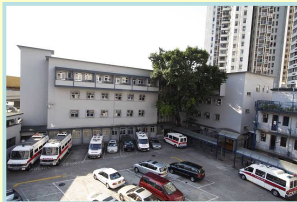
新翼 Annex Building
