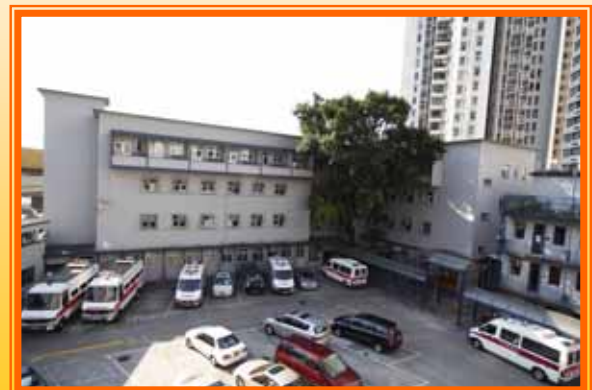
新翼 Annex Building
