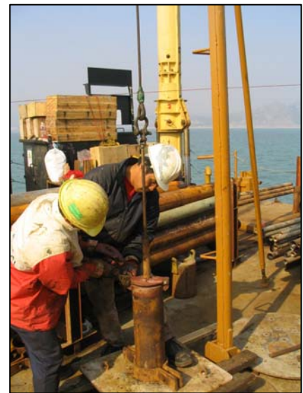
進行海上鑽探 Carrying out Marine Ground Investigation
